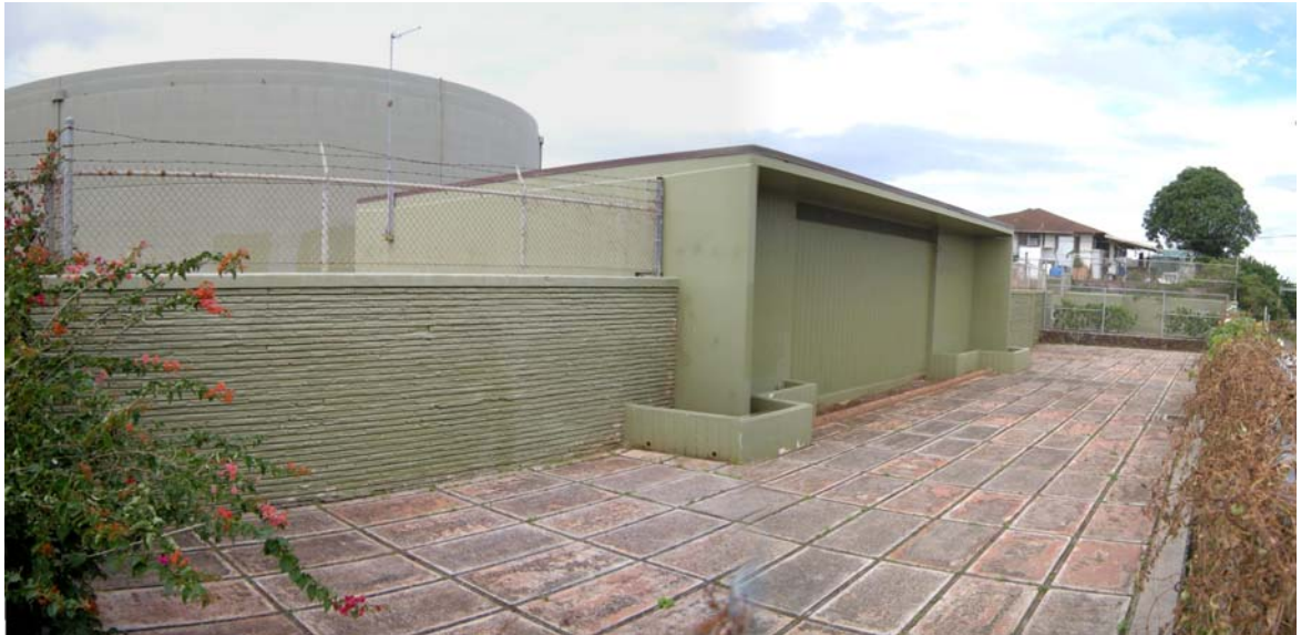
Figure 4-14: Āliamanu Water Pumping Station
