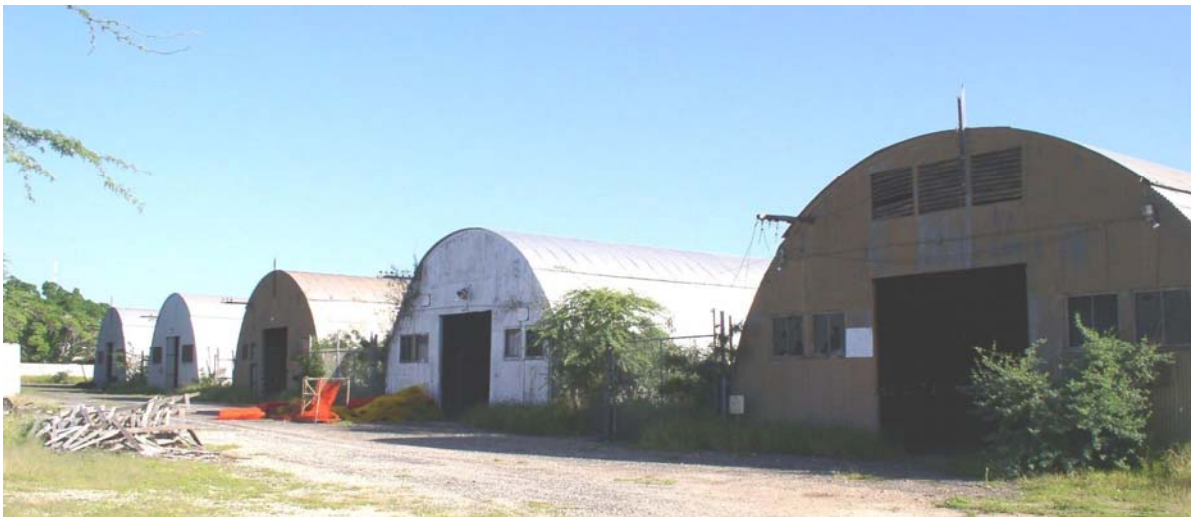
Figure 4-4: Facilities 1150, 1144, 1149, 1153 and 1152 – Quonset Hut Grouping, MCAS 'Ewa
