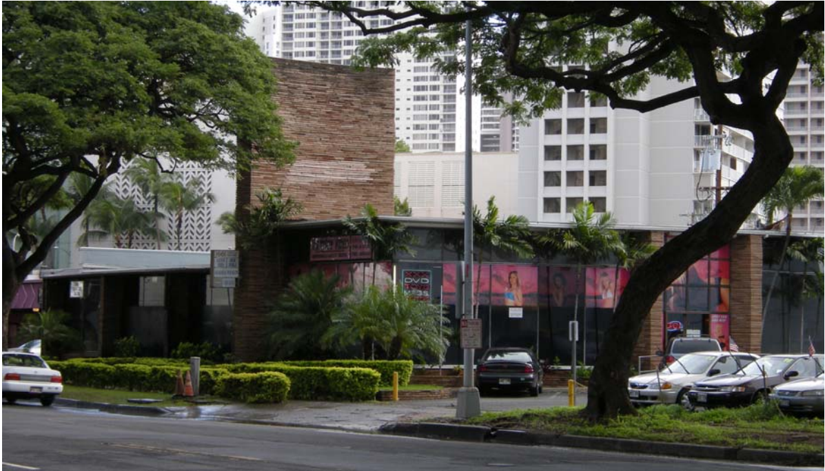
Figure 4-31: Boysen Paint Company Building
