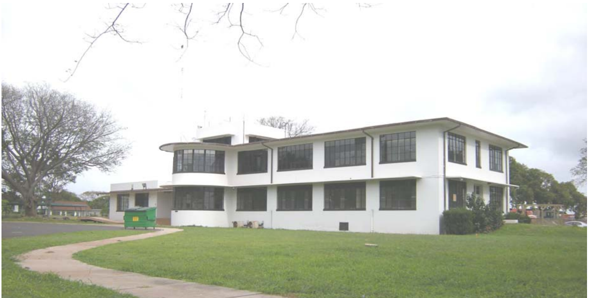
Figure 4-2: Facility 1—Administration Building
