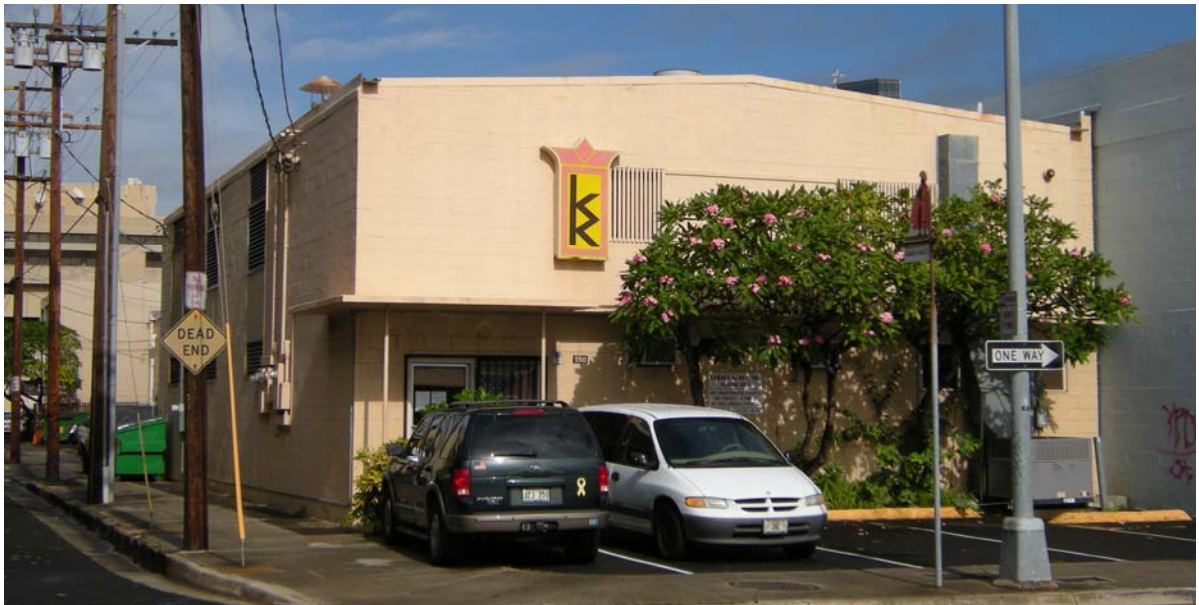
Figure 4-27: Kamaka Ukulele Building
