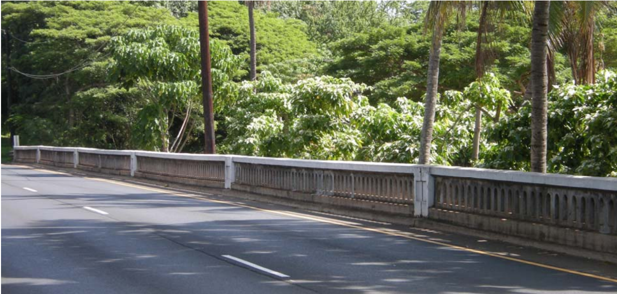
Figure 4-9: 1932 Waiawa Stream Bridge
