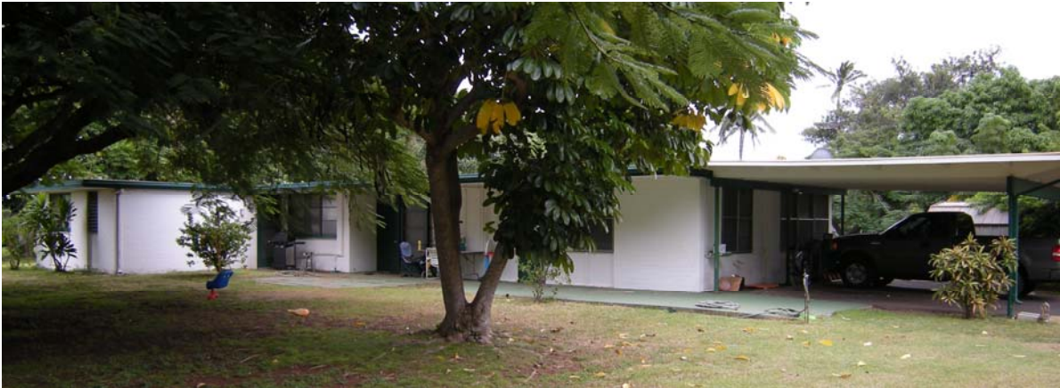
Figure 4-1: Example of 1953 House in NASBP Housing
