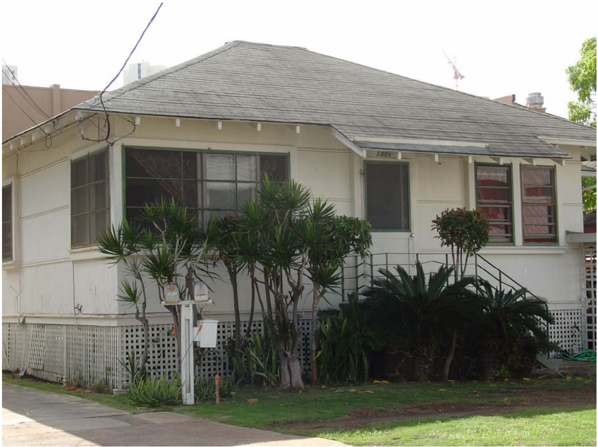
Figure 4-32: Wong House B (1911 Lime Street)
