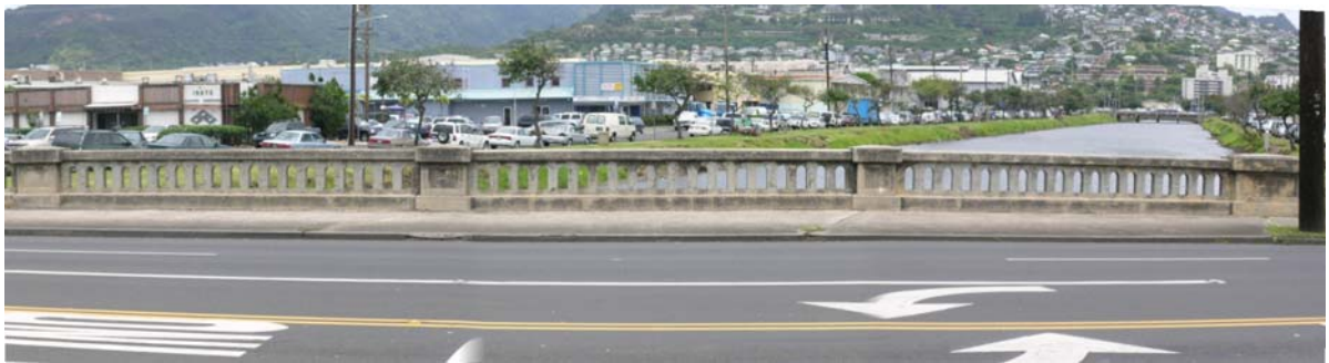
Figure 4-21: Bridge over Kapālama Drainage Canal
