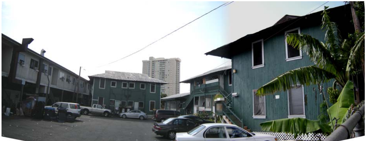
Figure 4-22: Tenements behind Tong Fat Building
