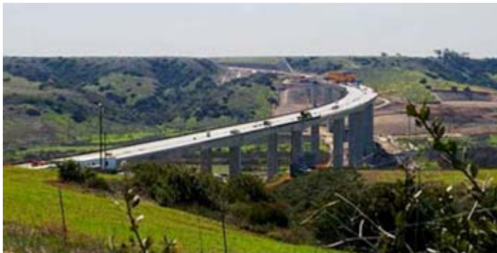
Otay Mesa River bridge near south end of South Bay Expressway
