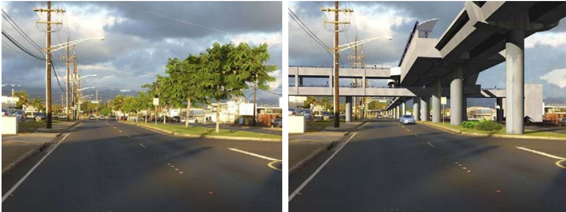
The above images are the before and after of the Waipahu rail transit station
