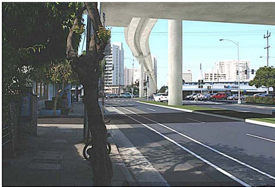
View from under the Varsity Theater rail station looking makai. The column widths are well understated a rail line 60 feet above ground. (City rendering)
