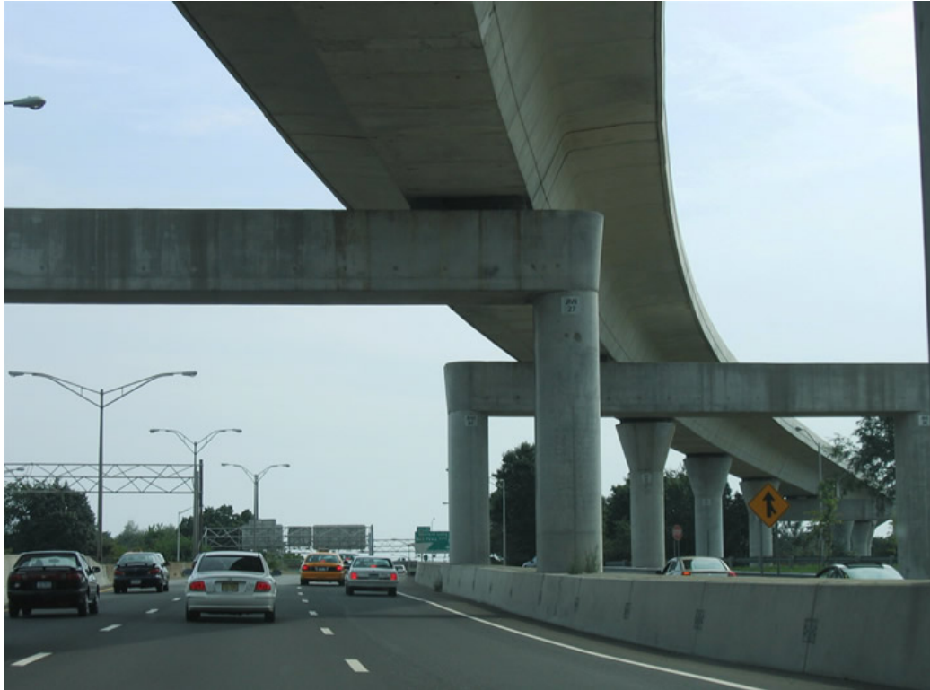
Photo of straddle bent supports under a New York highway. Notice that in the City rendering below how the sheer ugliness of straddle bent supports is minimized.
