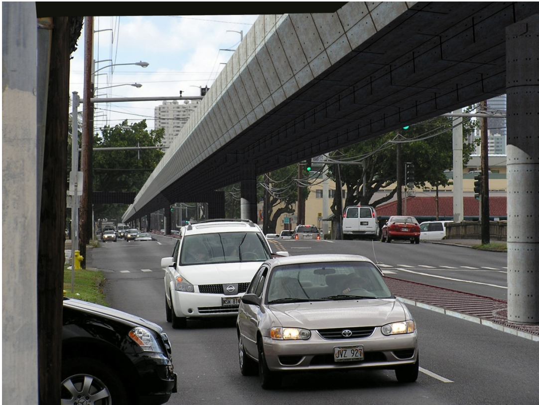
Our artists rendering of the sound mitigation panels to be used along Dillingham Blvd.
