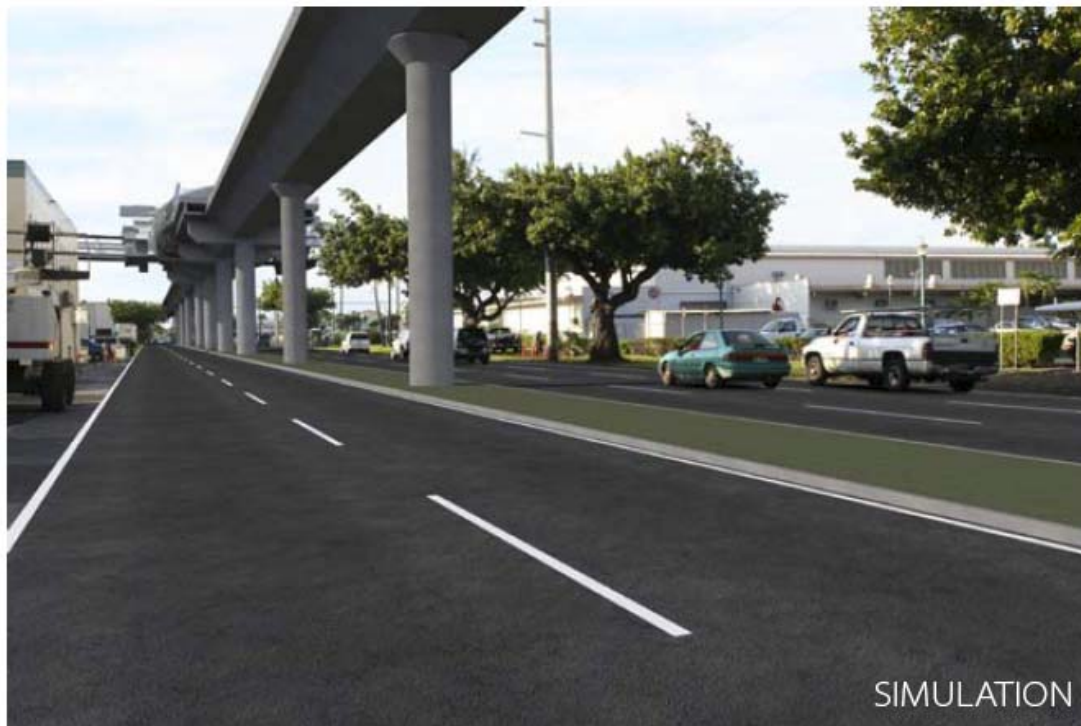
Figure 4-28 Viewpoint 12—Dillingham Boulevard near Honolulu Community College and Kapālama Station Area, looking 'Ewa
