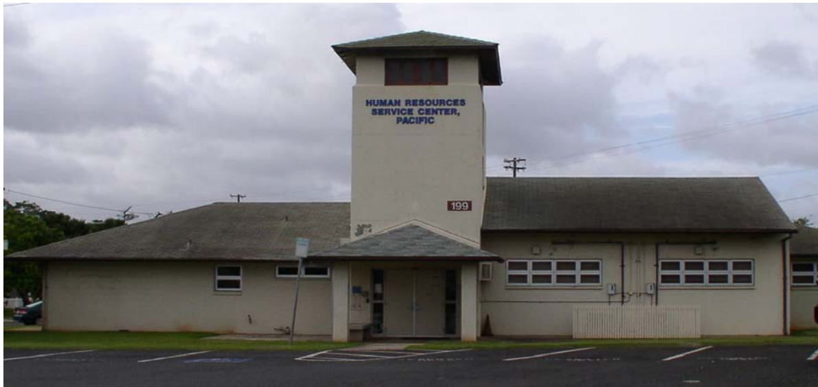
Figure 4-17: Rehabilitation Center/Former Navy Fire Station
