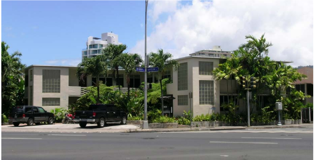
Figure 4-35: Fukumoto Apartments (2424 Kapi'olani Blvd.)
