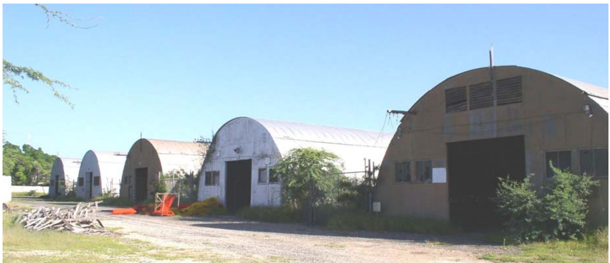
Figure 4-4: Facilities 1150, 1144, 1149, 1153 and 1152 – Quonset Hut Grouping, MCAS 'Ewa
