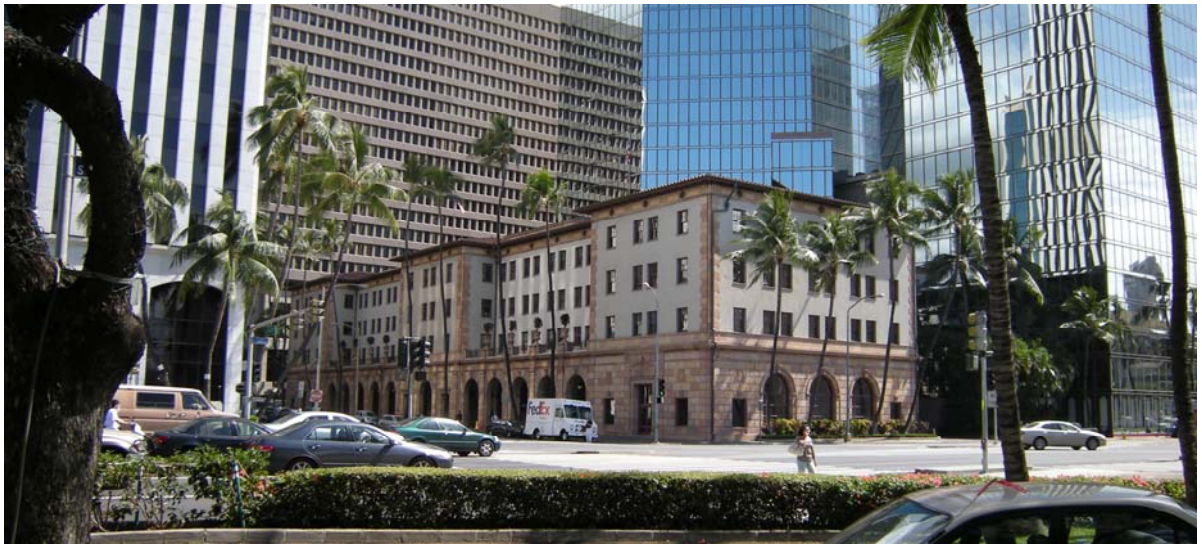
Figure 4-26: Dillingham Transportation Building
