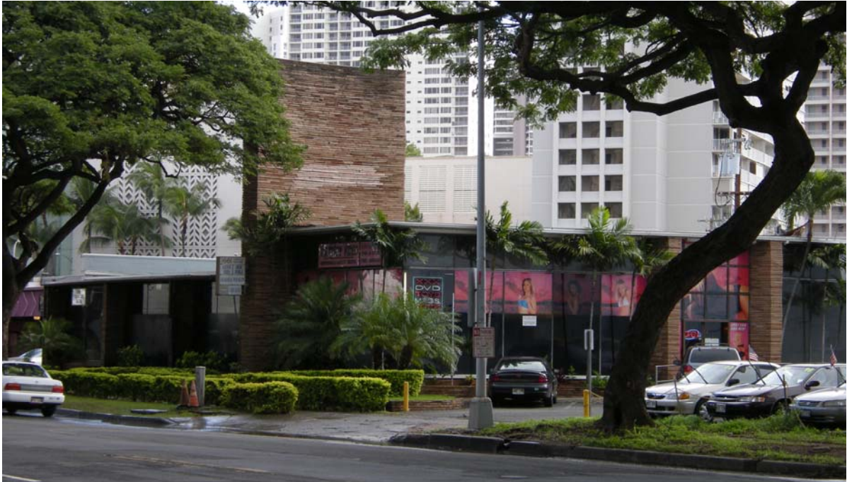
Figure 4-31: Boysen Paint Company Building
