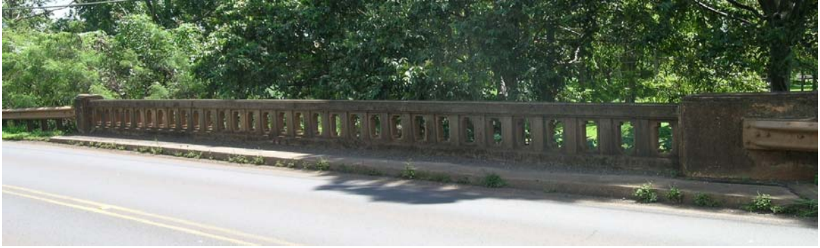
Figure 4-5: Farrington Highway Bridge over Hono'uli'uli Stream
