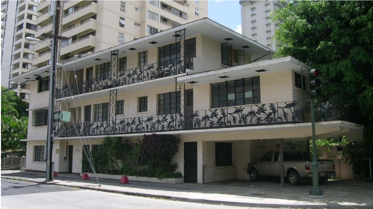
Figure 4-39: Ka'iulani Court Apartments (211 Ka'iulani Avenue)
