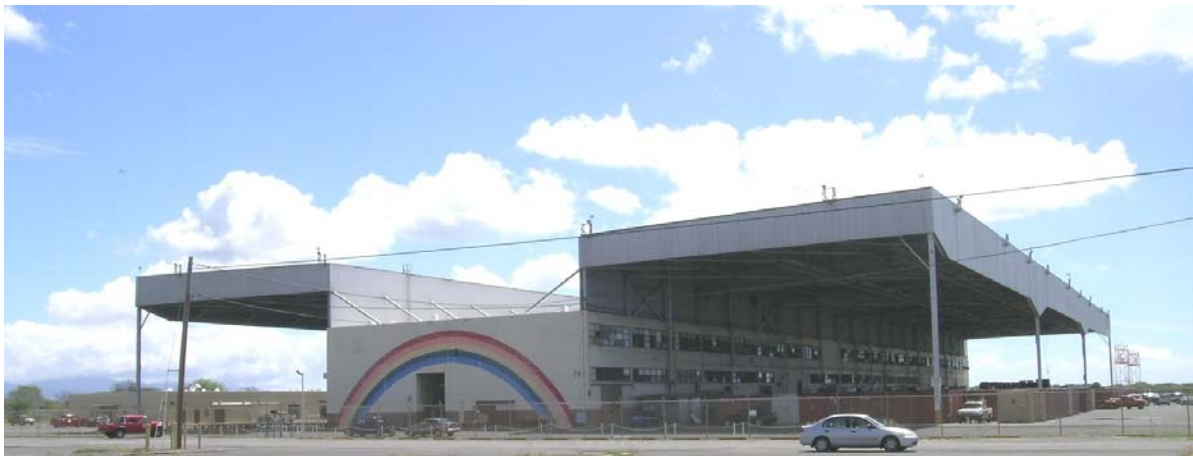
Figure 4-3: Facility 282—Cold War Hangar
