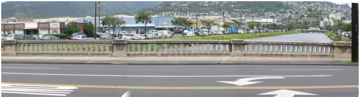
Figure 4-21: Bridge over Kapālama Drainage Canal
