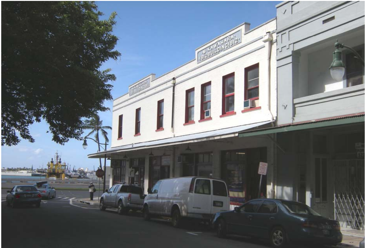
Figure 4-24: Kawahara Building with Honolulu Harbor in the Background
