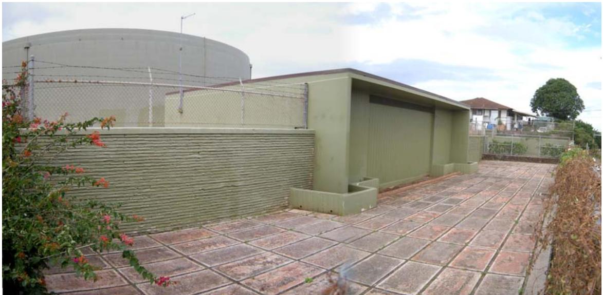
Figure 4-14: Āliamanu Water Pumping Station
