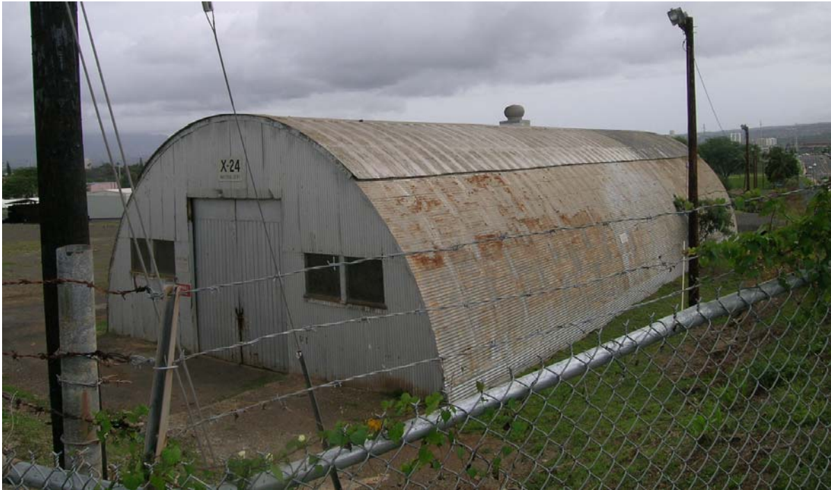
Figure 4-13: Facility X-24, Quonset Hut at the Navy Public Works Center
