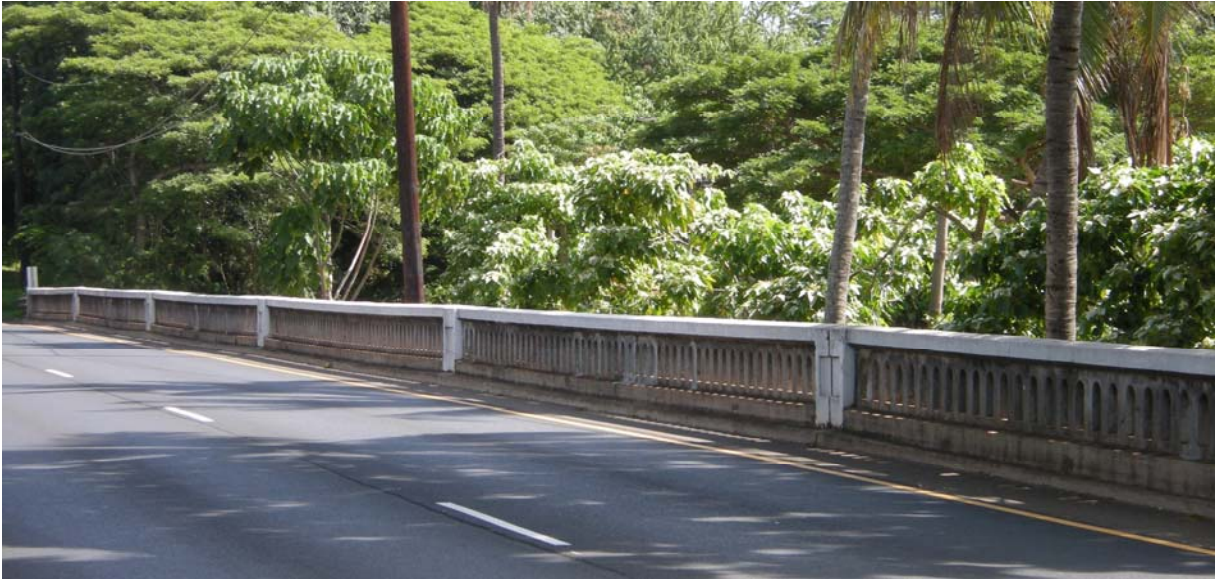
Figure 4-9: 1932 Waiawa Stream Bridge
