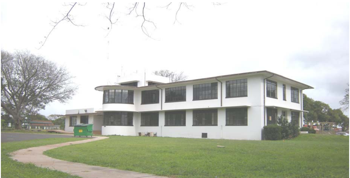
Figure 4-2: Facility 1—Administration Building
