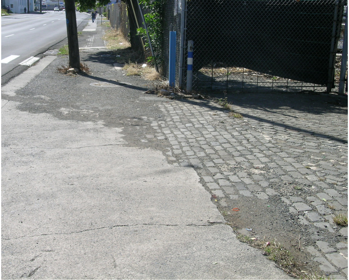
Figure 4-23: Basalt Street Paving alongside Iwilei Road at OR&L parcels
