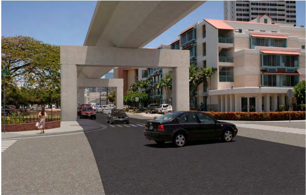
Figure 38. Existing View and Simulation of Elevated Guideway in Relation to the Mauka Boundary of Mother Waldron Neighborhood Park
