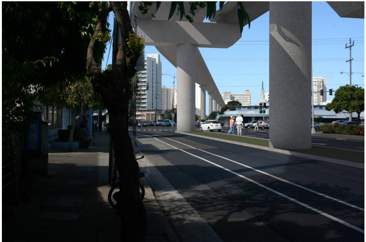
Figure 5-21: Viewpoint 4m Existing and Simulated Views—University Avenue near Varsity Place, Looking Makai
