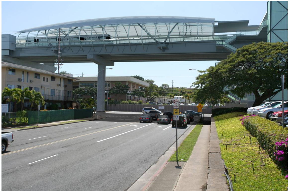
Figure 5-27: Viewpoint 3c Existing and Simulated Views—Ala Liliko'i Street/Salt Lake Boulevard Intersection near Ala Liliko'i Station, Looking Makai
