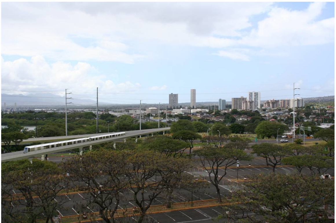
Figure 5-25: Viewpoint 3a Existing and Simulated Views—Aloha Stadium, Looking Mauka
