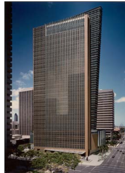
First Hawaiian Bank Center (tallest building on O'ahu, 1996, 420,000 sq. ft.)
