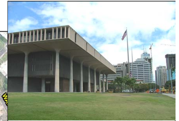
State Capitol Building
