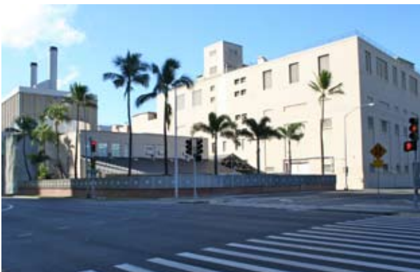
Figure 5-10 HECO Downtown Plant
