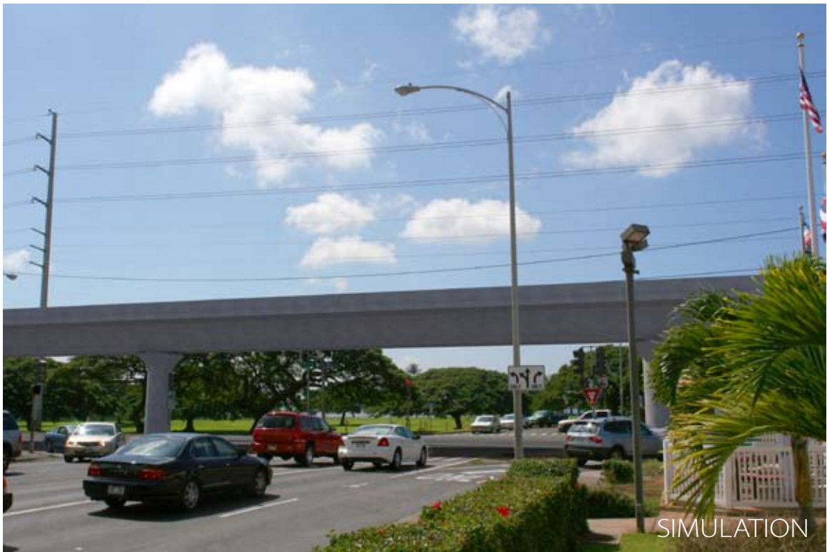
Figure 4-19 Viewpoint 3—Kamehameha Highway at Ka'ahumanu Street, looking Makai
