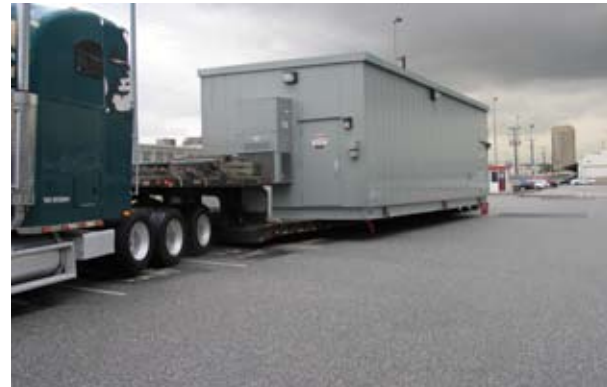
Figure 2-43 Installation of a Traction Power Substation
