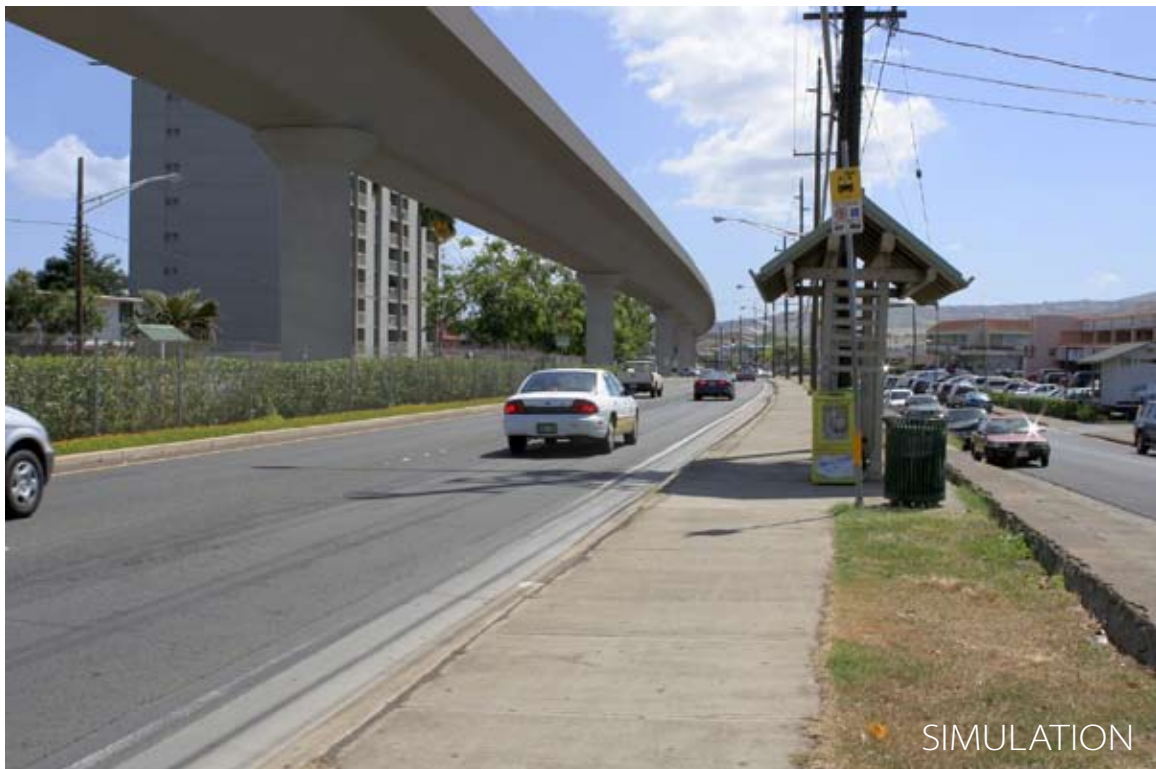
Figure 4-17 Viewpoint 1—Farrington Highway near Waikele Road, looking `Ewa
