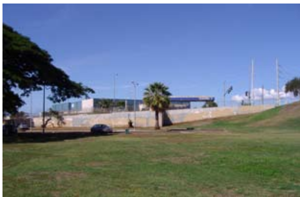
Figure 5-30 Āliamanu Park, looking makai. Guideway would be above retaining wall.
