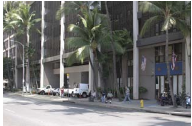
Figure 5-28 Parking Entrance at Harbor Square Building
