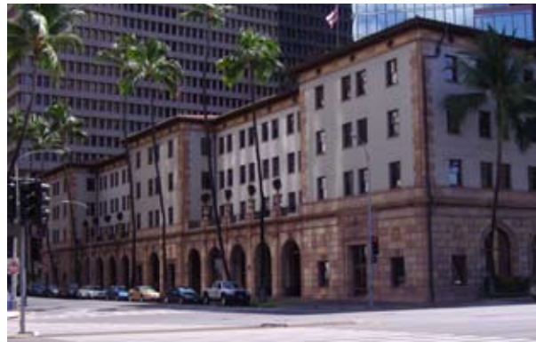
Figure 5-22 Dillingham Transportation Building
